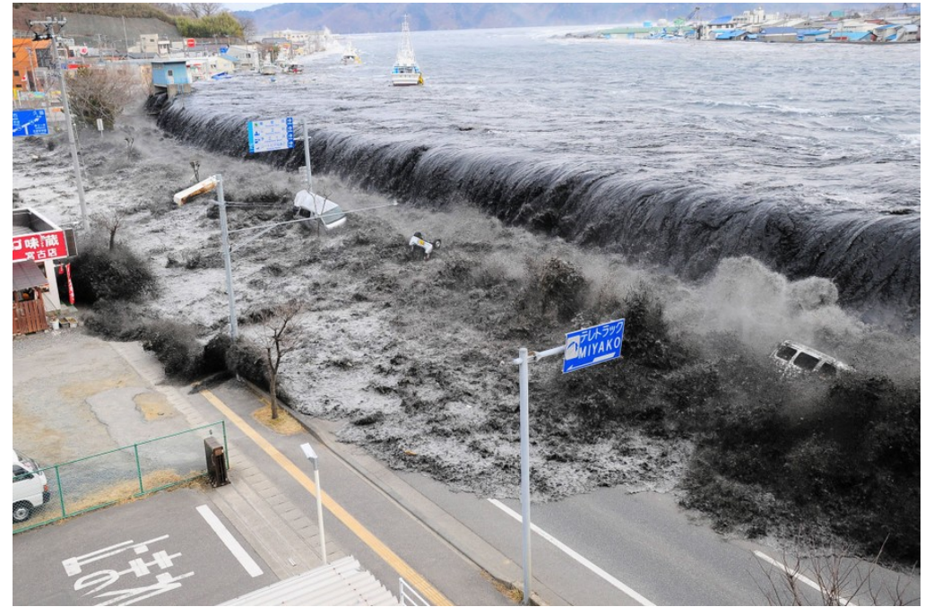
Coastal Road and Bridges: Miyako City (Iwate Pref) overtopping seawalls and flooding
