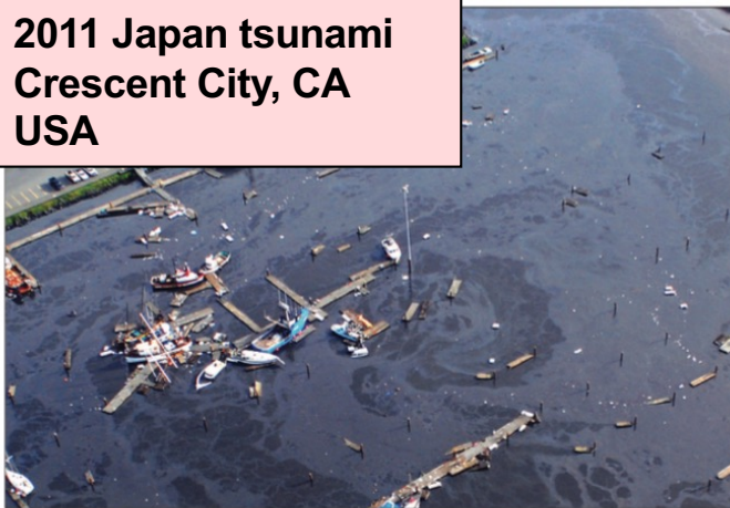
Crescent City, California boat harbor damage after the 2011 Japan tsunami. Strong wave currents entering the enclosed harbor (from top of photo) formed an eddy, which was left in the sediment swirls. The tsunami caused USD $55 million in damage to moorings and vessels in two dozen harbors in California. (Credit: R. Hiser and L. Dengler)
