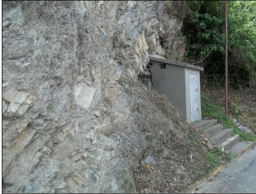
Figure 9. Real time seismological monitoring equipment. Source: SGC.
