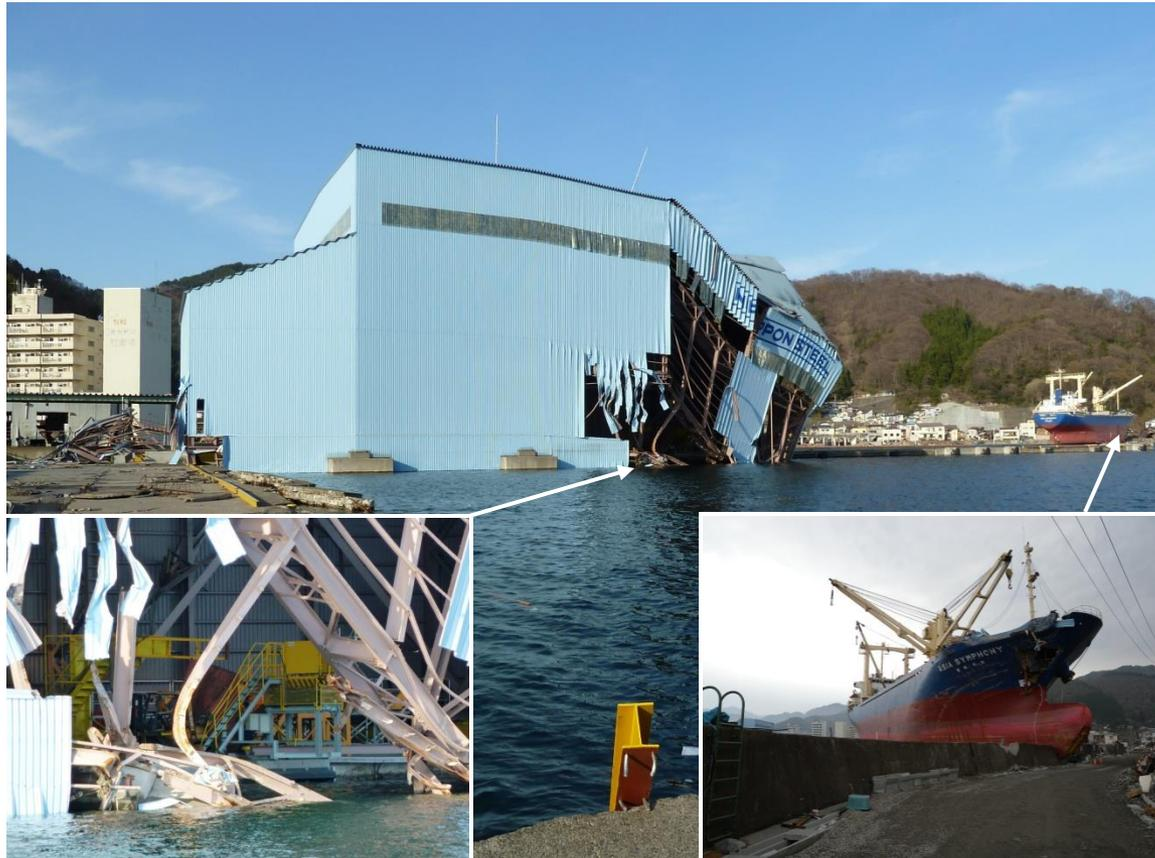
Ship impact damage to steel framed building on piled foundations in Kamaishi
