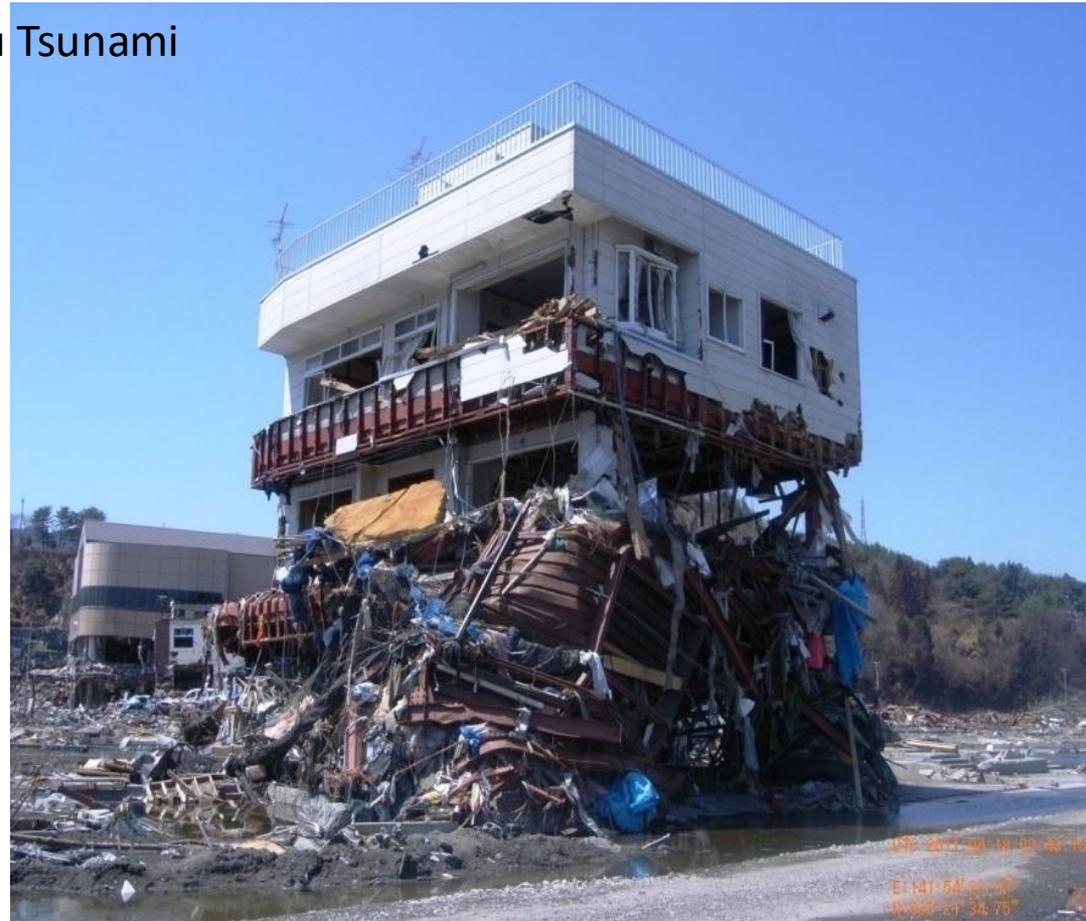
Three-Story Steel MRF with 5 meters of debris load accumulation wrapping
